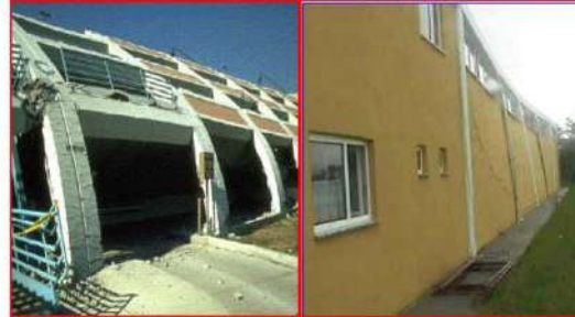
Fig. 4 Failure of irregular structures
