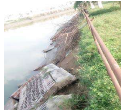
Fig.4 Depletion of rip-rap of bank
