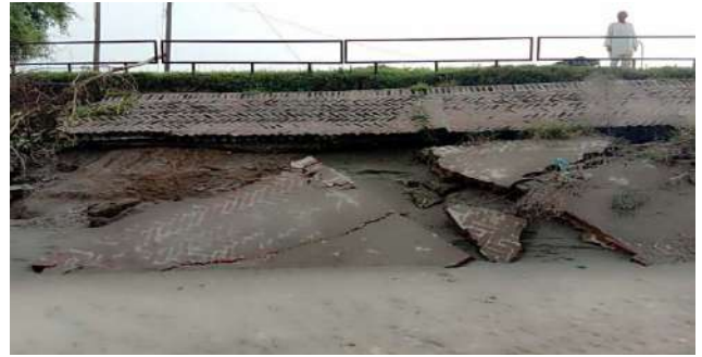
Fig.2 Destruction of banks of canal
